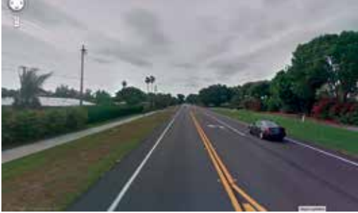
Current conditions along Gulf of Mexico Drive.
